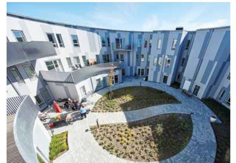
The inside of the figure eight encloses sunny and sheltered courtyards for residents.
